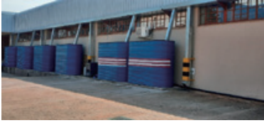
Water collection using the plant rooftop (YKK Southern Africa (Pty) Ltd.)
