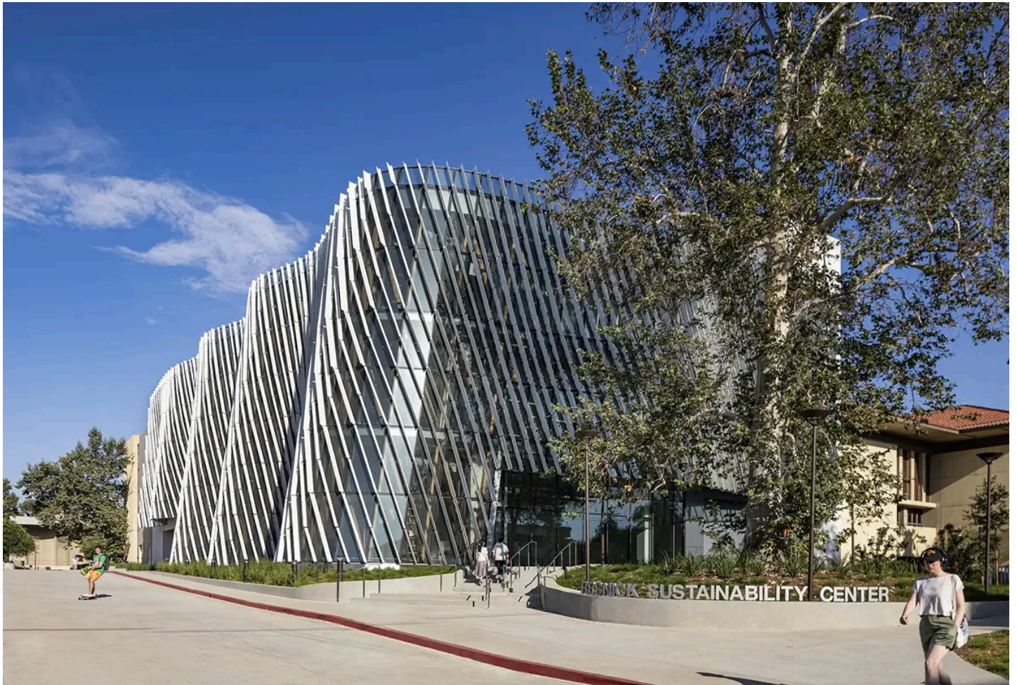
California Institute of Technology Resnick Sustainability Center, Pasadena, by Yazdani Studio of CannonDesign. Photo © Michael Moran
