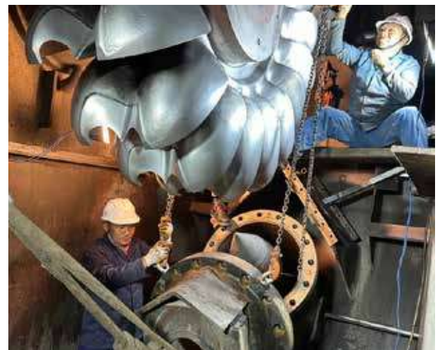
Replacement of Nozzle assemblies in Unit 1.
