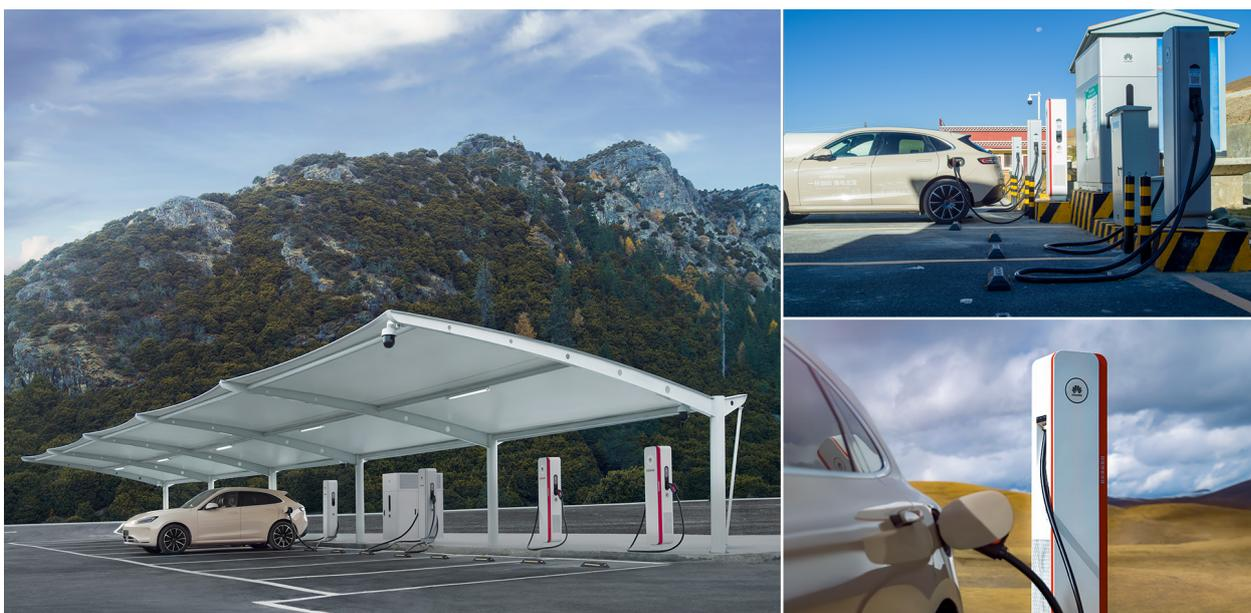
In September 2023, Huawei and its partners deployed fully liquid-cooled ultra-fast charging stations in Tianquan, Litang, and Sangdui, creating a Super Charging Green Corridor along the high-altitude G318 Highway. Heat dissipation is often a bottleneck in environments with low air pressure. Huawei has developed an innovative liquid-cooled technology that ensures ultra-fast high-power charging in these types of places. This technology can also improve long-term equipment reliability.
