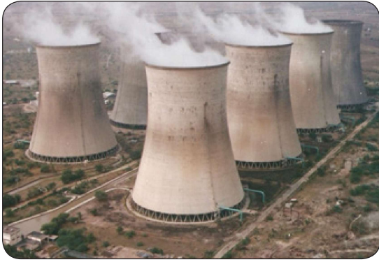
Raichur Cooling Towers
