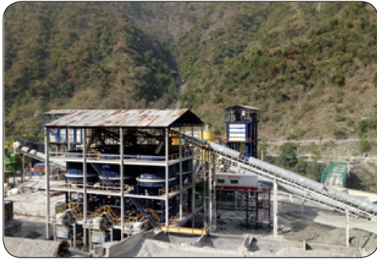
Temperature Controlled Concrete Production
