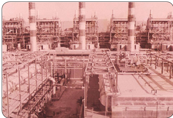
Tripoli West Thermal Power Station
