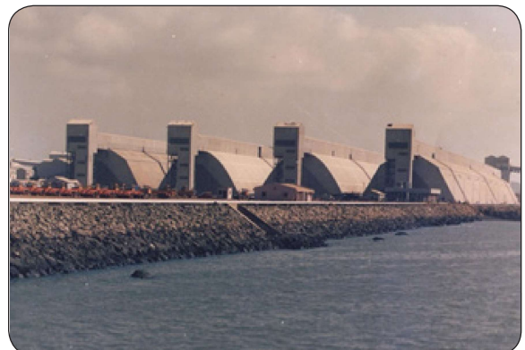
Nhava Sheva Bulk Handling Facility
