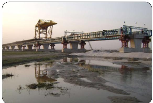
Camel Gantry for Segment Launching
