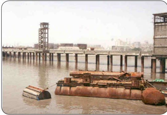
Kandla Oil Jetty
