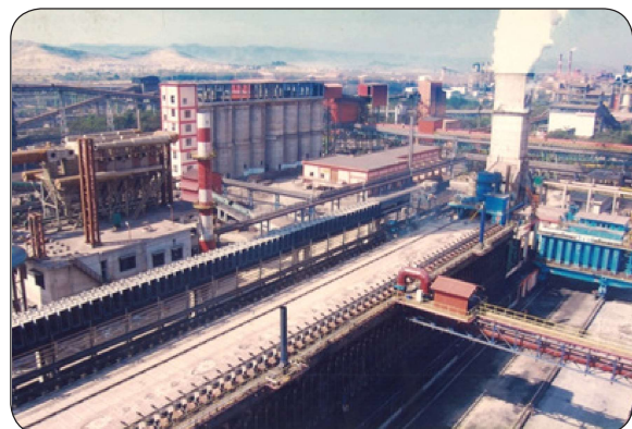
Vijay Nagar Steel Plant
