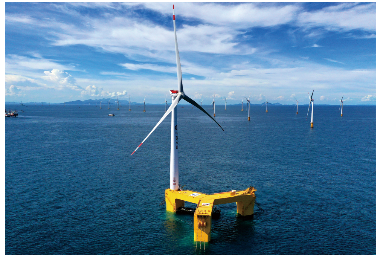
● CTG Leader, the first floating offshore wind turbine — wind farm platform in China
