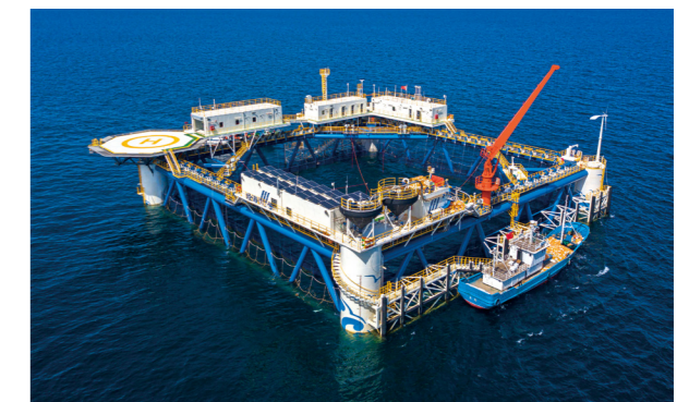
● JING HAI 002, a deep-water intelligent fish farming installation
