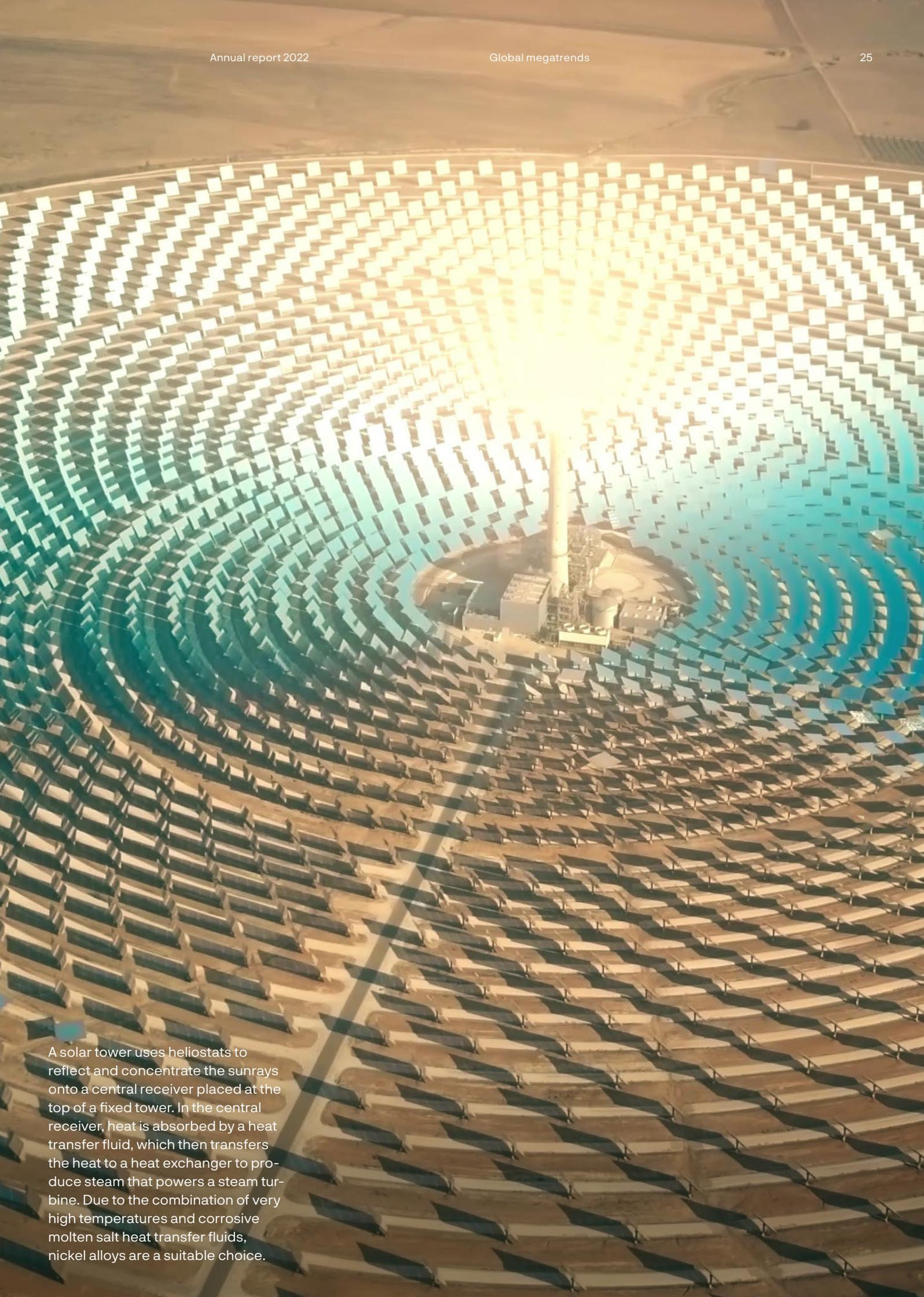
A solar tower uses heliostats to reflect and concentrate the sunrays onto a central receiver placed at the top of a fixed tower. In the central receiver, heat is absorbed by a heat transfer fluid, which then transfers the heat to a heat exchanger to produce steam that powers a steam turbine. Due to the combination of very high temperatures and corrosive molten salt heat transfer fluids, nickel alloys are a suitable choice.
