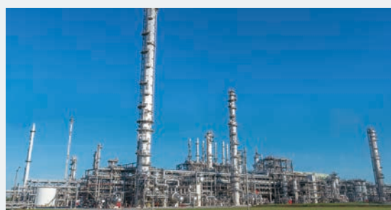
Shintech's ethylene plant that started operations in 2020 (Louisiana, USA)
