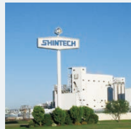
Shintech Freeport Plant (Texas, USA)
